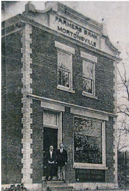
The historic bank in Mortonsville
